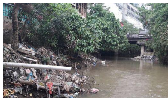
Figure 7: Waste Stacks and Household Disposal Pipes
