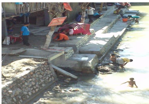
Figure 11: Wall of the River Water Buffer Embankment
