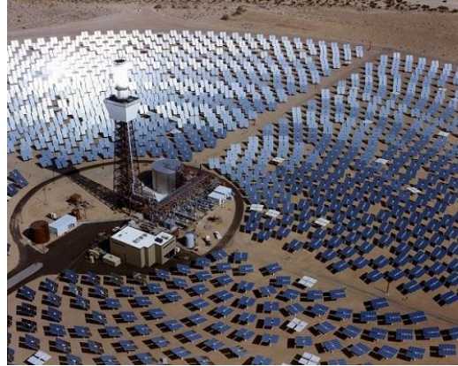
Fig. 5. CSP Power tower system requires water to cool down.
