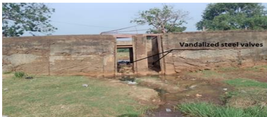
Figure 5: Two vandalized metal valves at the dam of the Founkama micro-dam (Photo. Babilas Hountondji, 2026).
