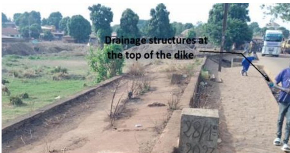
Figure 7: Drainage structure at the top of the micro-dam of Founkama (Photo. Babilas Hountondji, 2026).
