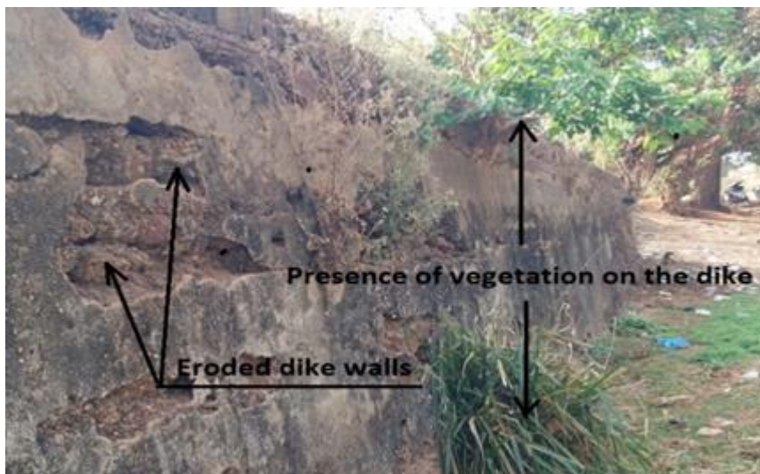
Figure 9: Vegetation presence and degradation observed on the Founkama micro-dam (Photo. Babilas Hountondji, 2026)
