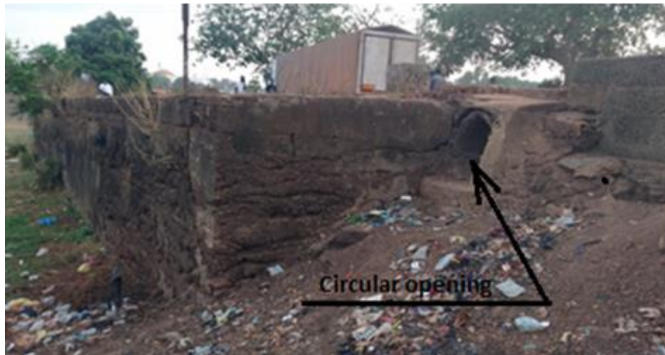
Figure 6: Circular evacuation opening at the level of the dike of the Founkama micro-dam (Photo. Babilas Hountondji, 2026).
