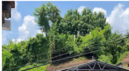
Figure 3. The existence of bioengineering engineering slope retaining in landslide-prone locations
