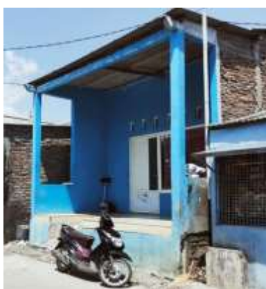
Figure 4. The foundation of the house is higher than the ground.
