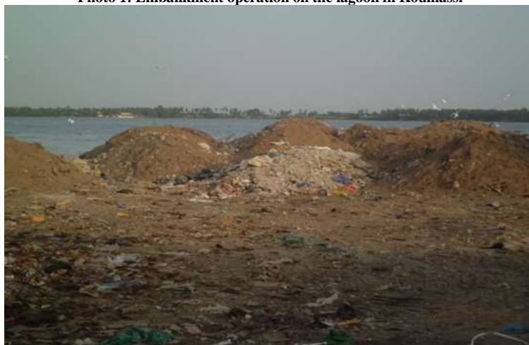
Photo 1: Embankment operation on the lagoon in Koumassi
